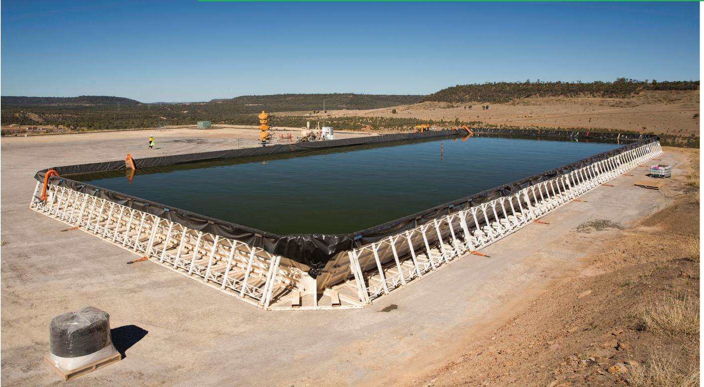
MPC Kinetic has developed patented FlexiPond technology to assist with above ground oil field fluid management, significantly reducing excavation costs.
